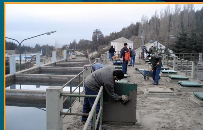
Ash can enter sand filters both by direct airfall and through intakes. Cleaning of filter beds may create heavy additional labour demands, such as at Bariloche's main water treatment plant following the June 2011 eruption of Cordón Caulle volcano, Chile, which deposited ~30-45 mm of ash across the city.
