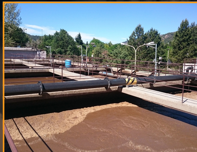
Biological reactors at the municipal wastewater treatment plant at San Martin de los Andes, Argentina, continued to function without problems despite receiving 2 cm of ashfall from the 2015 eruption of Calbuco volcano, 165 km away in Chile. This was partially because the town's storm drains and sewers are well separated, so very little ash entered the plant in raw wastewater. Photo credit: Daniel Blake
