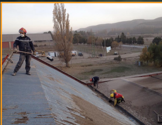
Volunteer firefighters work to clean ash from roofs in the town of Junin de los Andes, Argentina. Following the April 2015 eruption of Calbuco volcano in Chile, 200 km to the southwest, approximately 3 cm of fine andesitic ash fell across the town of Junin. Photo credit: Bomberos Voluntarios, Junin de los Andes.
