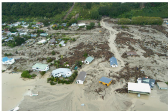
e) Inundation of buildings, Matatā 2005
