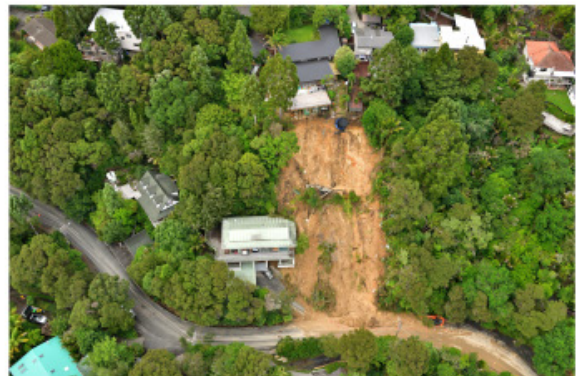
d) Undermining and inundation of buildings, Auckland 2023
