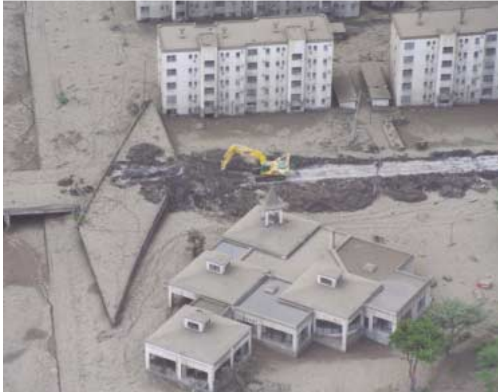
(Left) Lahar debris filled the ground floor of these apartments in the Toya Hot Spring area, Abuta Town, Hokkaido. Courtesy of Professor Hiromu Okada, Hokkaido University
