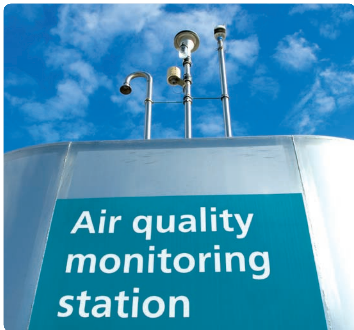
Air quality monitoring station in Lower Hutt, providing daily air particulate measurements
