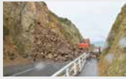
P41 Landslip at Pass of Branda, Seatoun, Wellington – Will Ries
