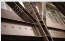
P14 Quake strengthening, Wellington – Gerry le Roux, ScienceLens
