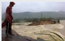
P3 Ruptured irrigation dam in Vietnam – Ngoc Minh
