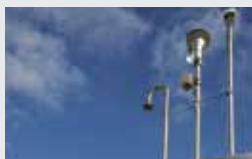
P1 Wellington Regional Council air monitoring station in the capital – Kate Whitley, GNS Science
