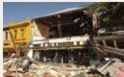
IC CBD damage, Christchurch earthquake – Margaret Low, GNS Science
